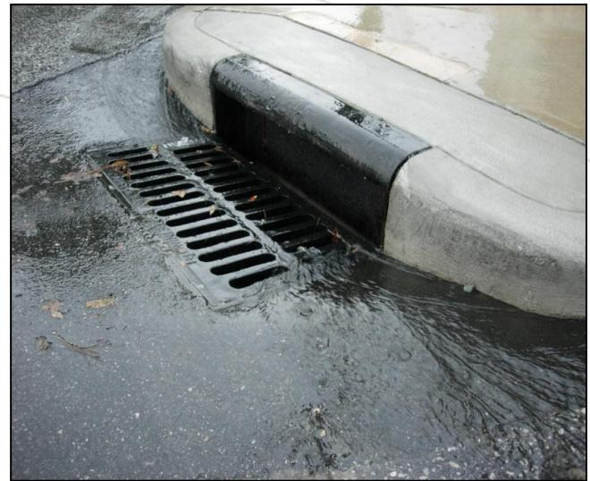
Impervious surfaces decrease infiltration, increase runoff and allow pollutants to accumulate. Runoff determines size of storm sewer system.
