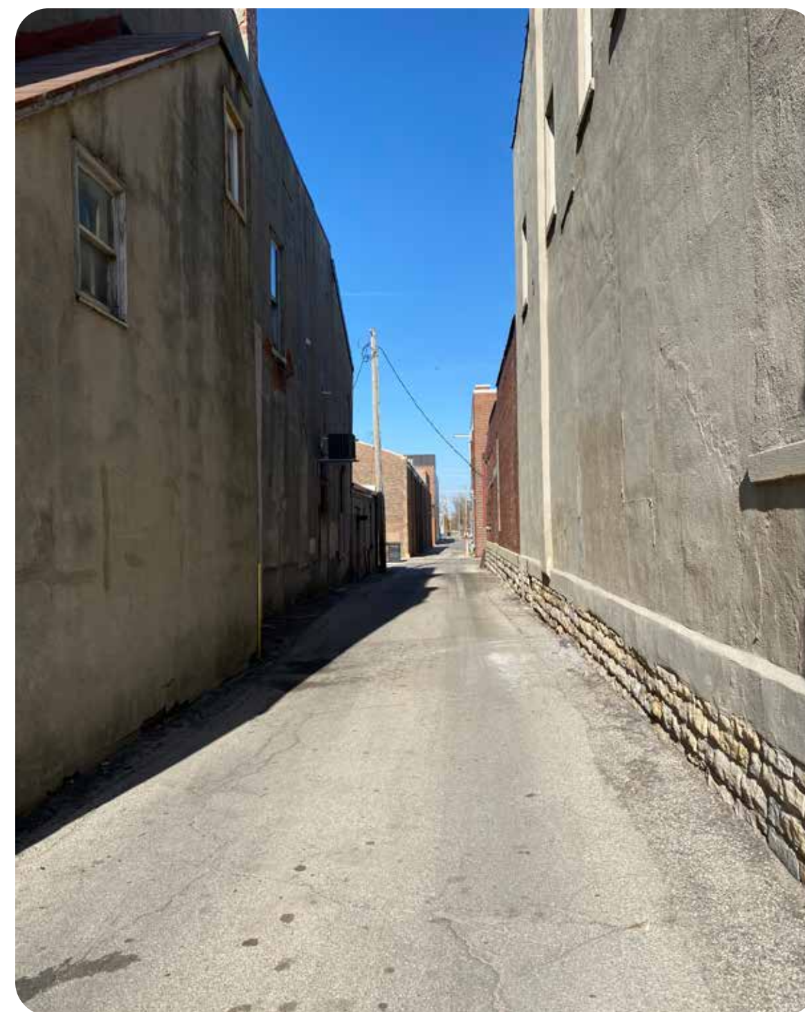
EXISTING ALLEY W/ NO IMPROVEMENTS
