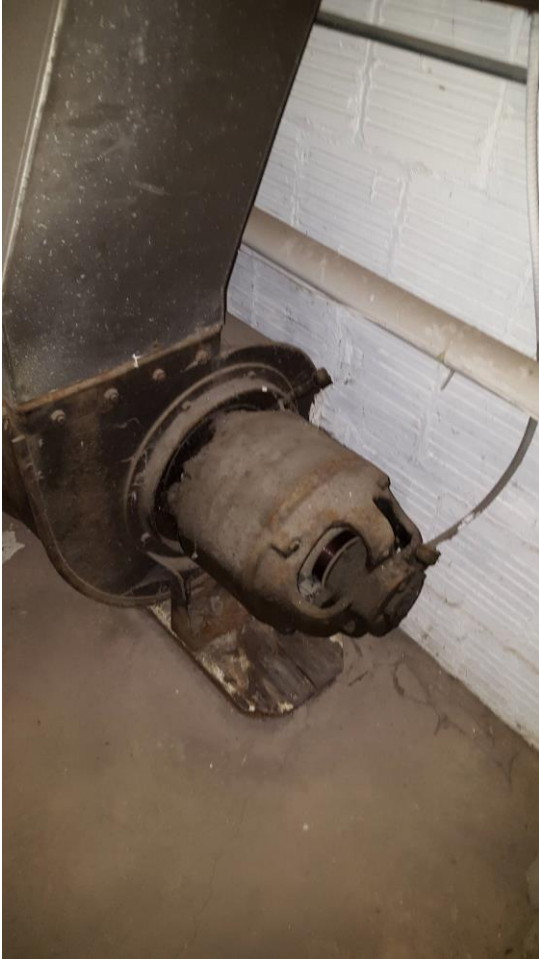
Figure 5: Antiquated restroom exhaust fan
