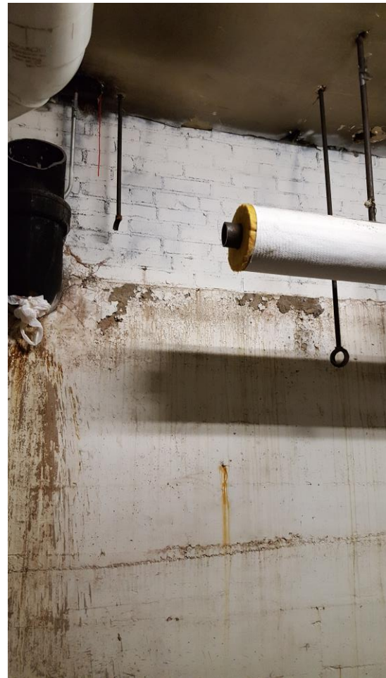
Figure 2: Cut steam piping
