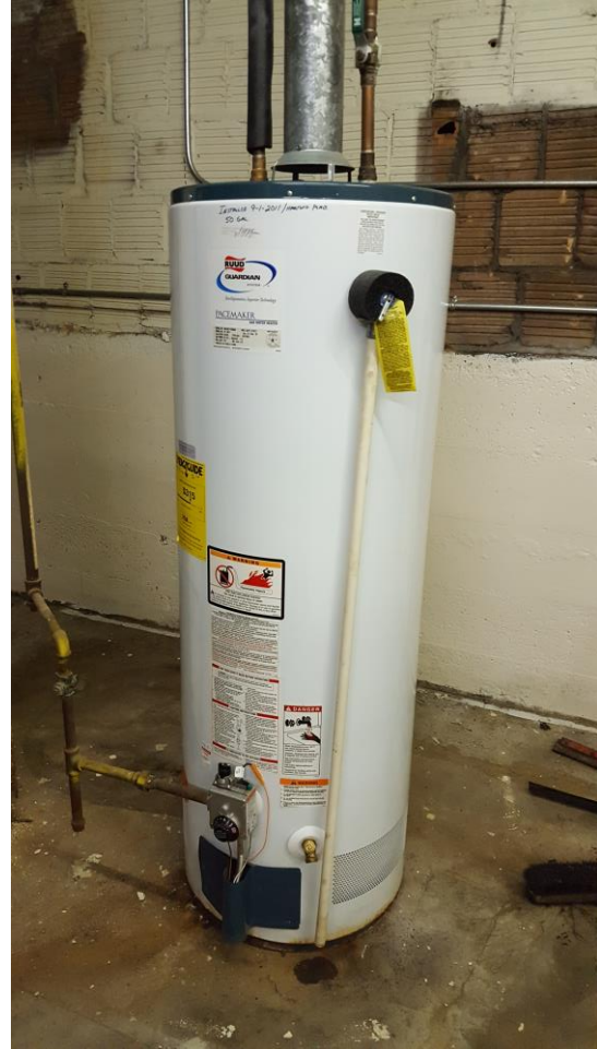
Figure 10: Natural gas hot water heater
