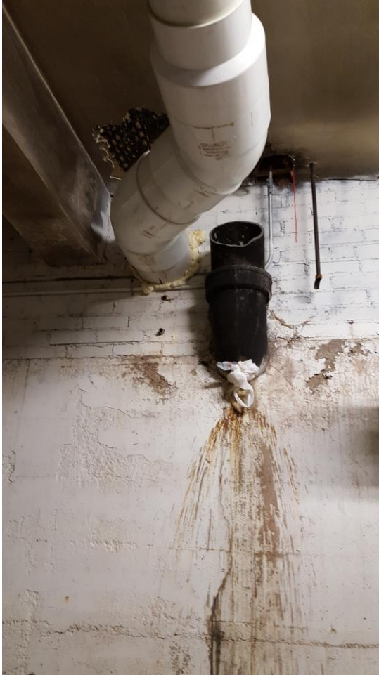
Figure 9: Updated PVC piping next to out-of-service piping
