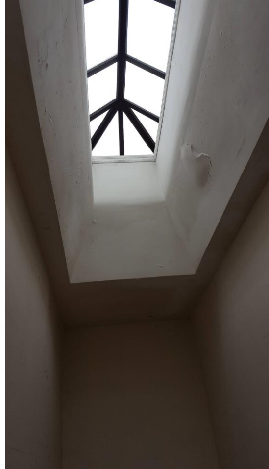
Figure 16: Water damage under skylight
