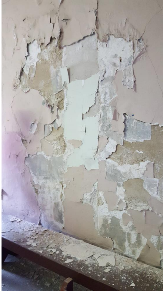
Figure 17: Water damage on East wall, second floor
