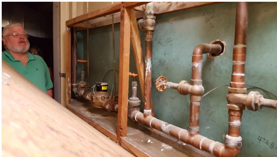
Figure 12: Domestic water piping and water meter
