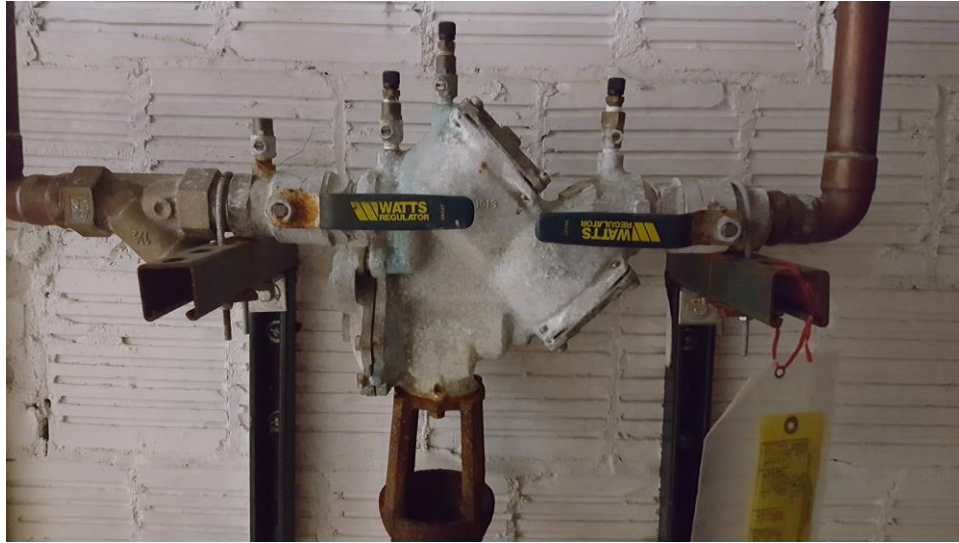
Figure 11: Backflow preventer
