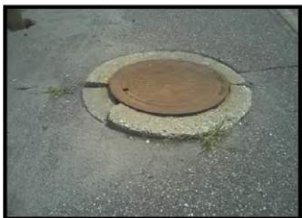
Traffic Signal Handhole
